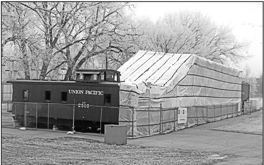
UP “Big Boy” 4004 is encapsulated in preparation for asbestos removal on February 9, 2018. The UP caboose (on a frame, without trucks) is privately owned and is used as a warming shelter and a place for changing in and out of proper safety apparel required for asbestos removal workers.
